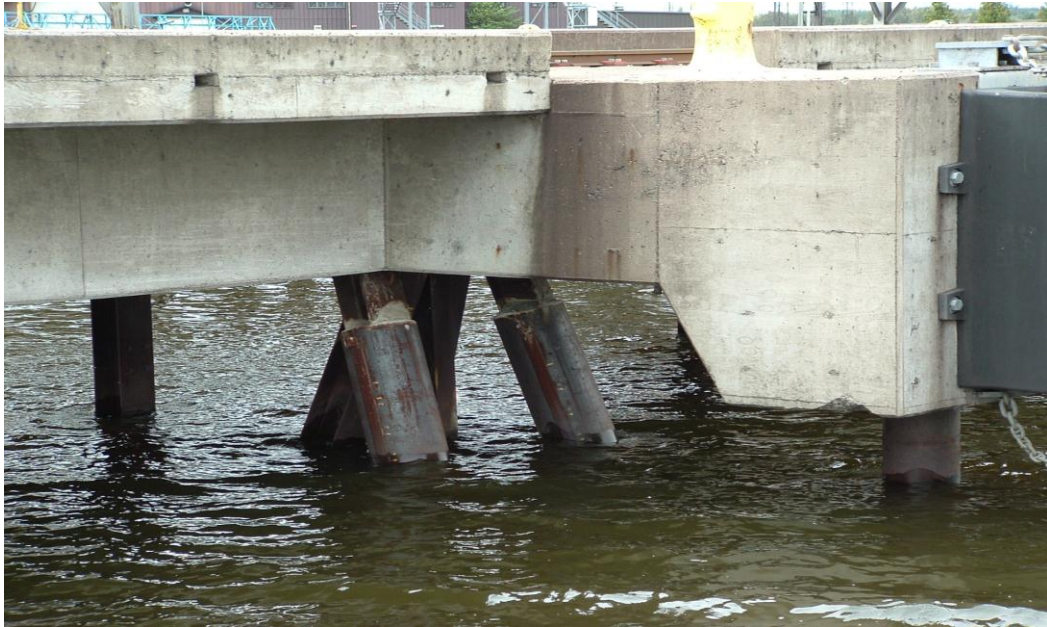
Photo 3. H-Pile Jacketing Repair
